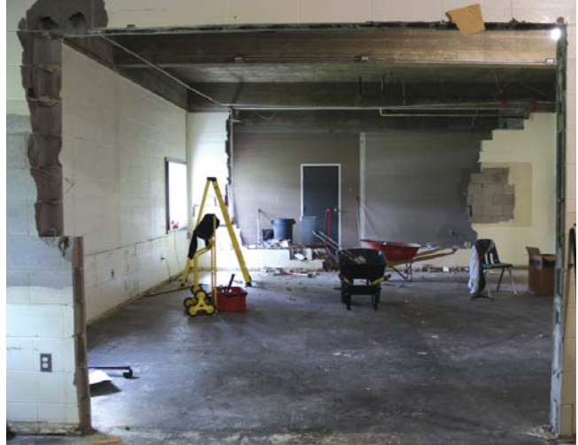
McNaughton High School begins demolition in Home Ec lab.
