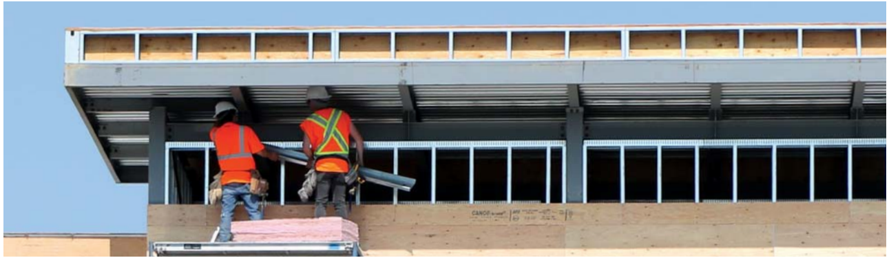
Two workers working on Moosomin's Co-op grocery store on Thursday.
