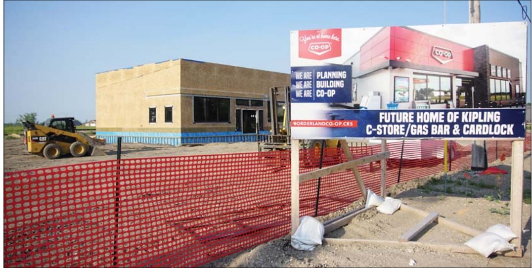
Construction is progressing on the Borderland Co-op Gas Bar in Kipling.
