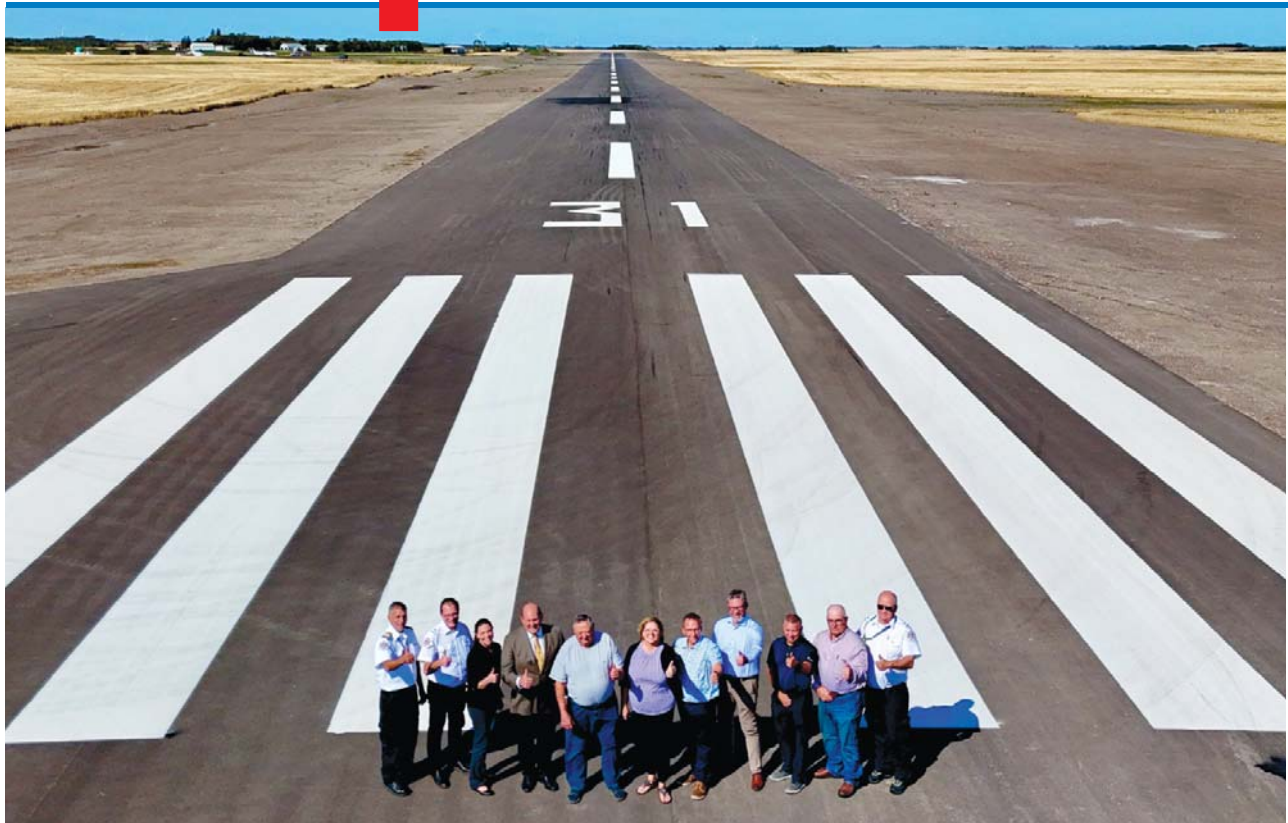
The new 5,000 foot runway at Moosomin Airport. Saskatchewan Highways Minister Lori Carr visited Moosomin Tuesday to see the expanded airport. This view from the south end of the runway shows the scale of the project.
