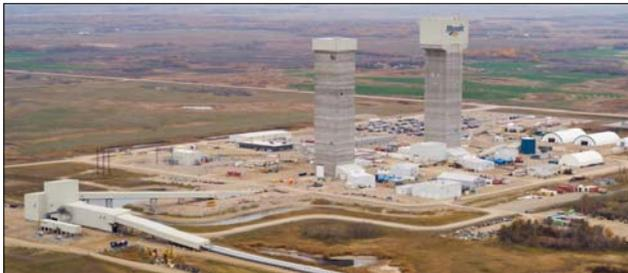
K3 came fully online in 2022, and its design and technology make Mosaic's Esterhazy facility the world's most advanced and largest potash operation. The early development of K3 started in 2009, with the sinking of the shaft beginning in 2011, and crews successfully reaching ore level in 2017. The cost to build K3 was \$2.9 billion.
