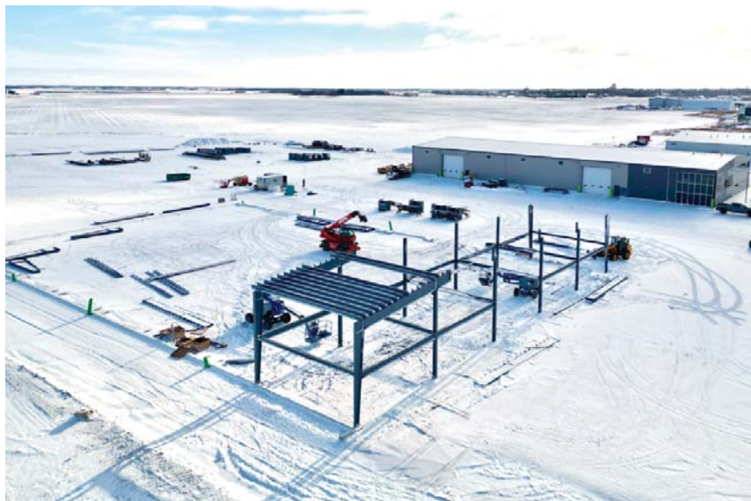
The IJACK expansion underway at their facility north of Moosomin.
