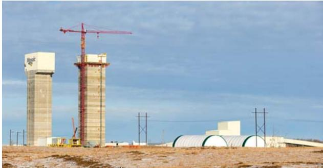
When the south shaft headframe is fully operational in March 2022, it will double the hoisting capacity at K3. Each shaft will have 36,000 tons per day hoisting capacity—for a total of 72,000 tons.
