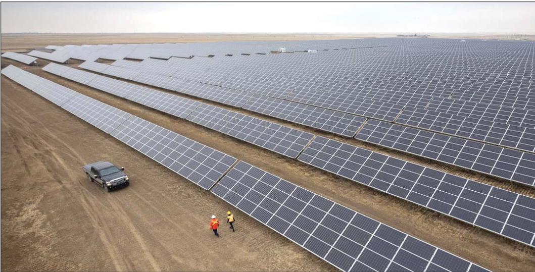
Enbridge's first solar self-power project in Canada between Lethbridge and Medicine Hat. Alberta Solar One, as it's known, supplies a portion of power to the Enbridge Mainline pipeline network, which includes the Line 3 replacement pipeline. The facility features 36,000 solar panels and has a capacity of 10.5 megawatts, equivalent to meeting the energy needs for about 3,000 homes and offsetting 12,000 tonnes of carbon annually.
