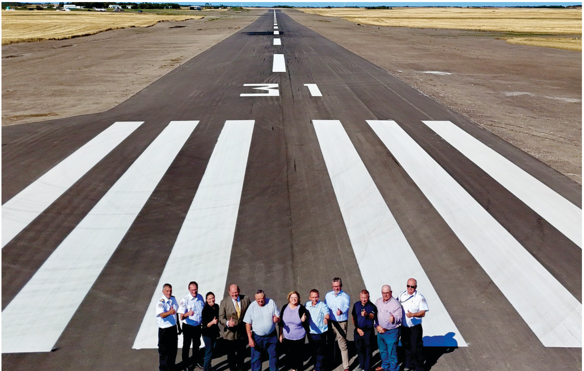
The new 5,000 foot runway at Moosomin Airport. Saskatchewan Highways Minister Lori Carr visited Moosomin recently to see the expanded airport. This view from the south end of the runway shows the scale of the project.
